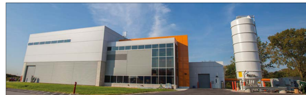
Fig. 1. The new MC-1 building at Fermilab, where the muon g-2 storage ring is being reassembled in the larger part to the left. The part to the right houses the counting room, electronics, etc, with cryogenics services further right. (Image credit: Fermilab.)
